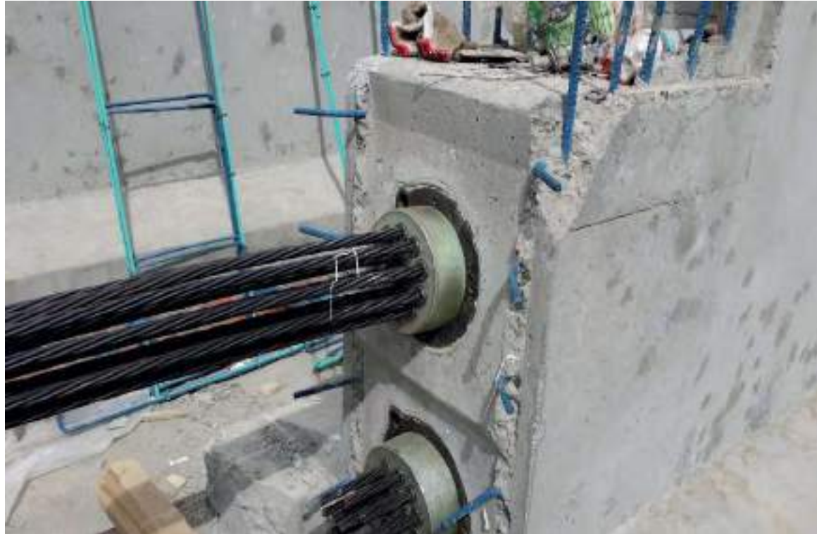
Abha Bridge – Post Tensioning Bridge Girder
