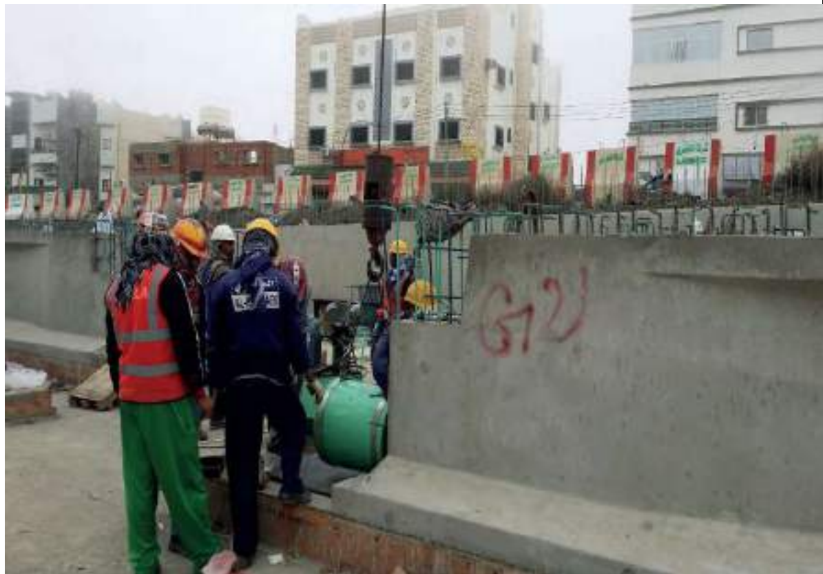
Abha Bridge – Post Tensioning Bridge Girder
