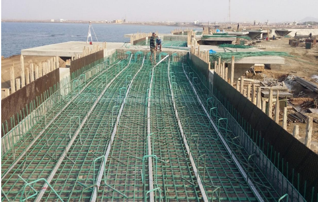
Fishing Bridge, Harida Aseer Province – Post Tensioning of Bridge
