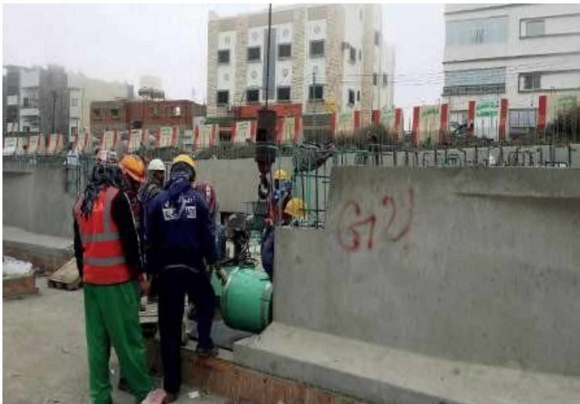
Abha Bridge – Post Tensioning Bridge Girder
