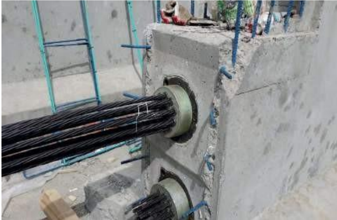
Abha Bridge – Post Tensioning Bridge Girder
