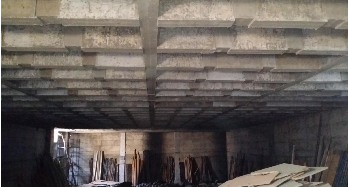
Fakeeh Theater Roof, Makkah – Post Tensioning of Slab
