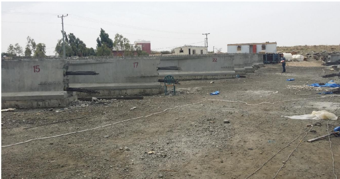
Al Ma'arid, Abha Underpass – Post Tensioning Bridge Girder
