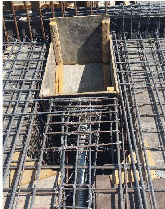
Fakeeh Theater Roof, Makkah – Post Tensioning of Slab
