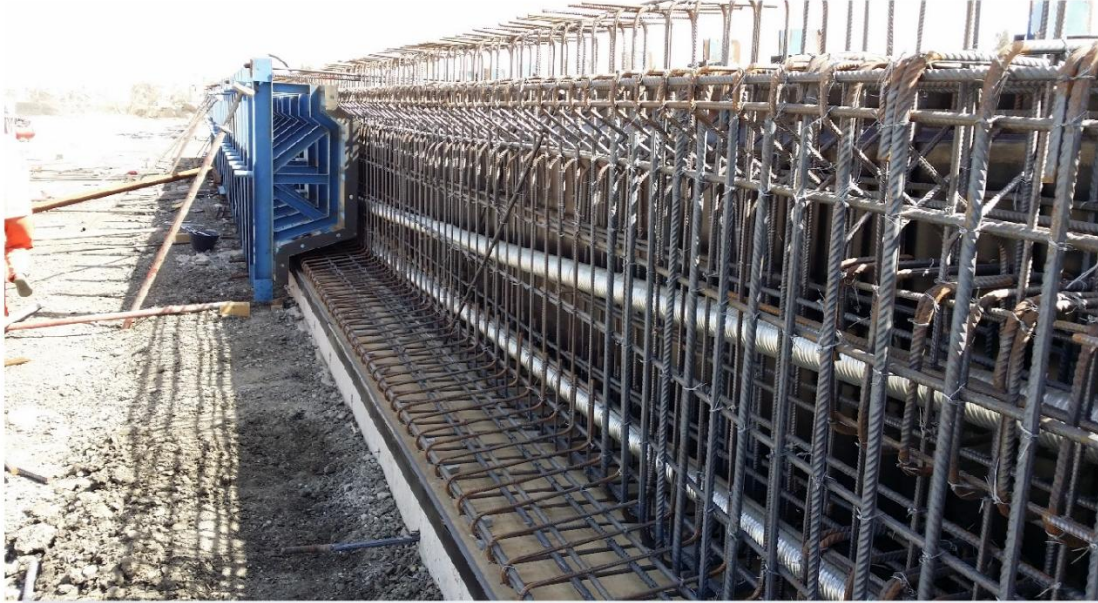
Al Ma'arid, Abha Underpass – Post Tensioning Bridge Girder
